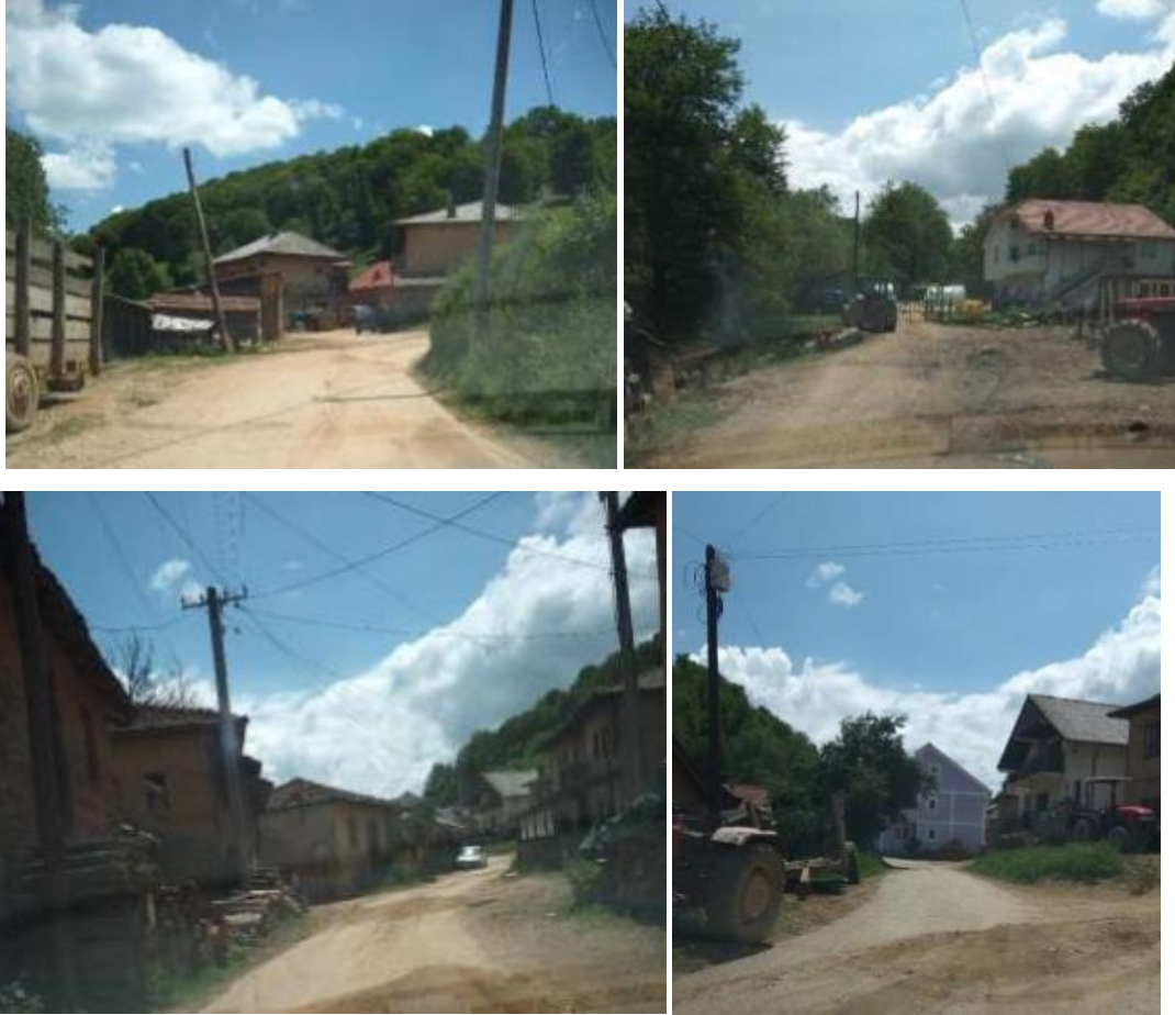
Figure 6 Current situation of the project area in village Dvoriste
